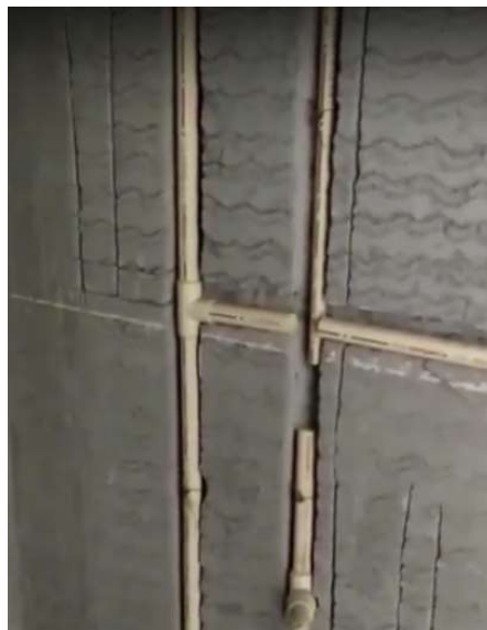
Plumbing conduits & boxes placed in AAC wall.
