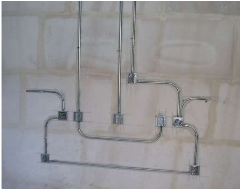
Electrical conduits & boxes placed in AAC wall.
